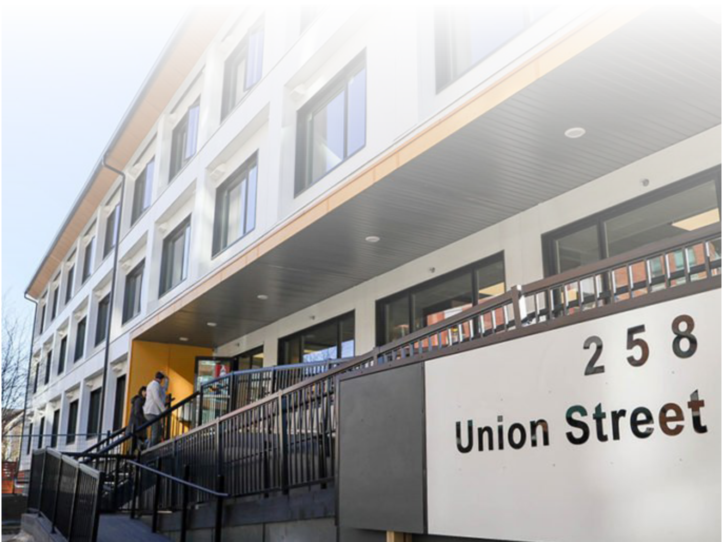
Hogan's Alley Society currently offers 52 affordable units in temporary modular housing next to Vancouver's Chinatown and Strathcona neighbourhoods.
